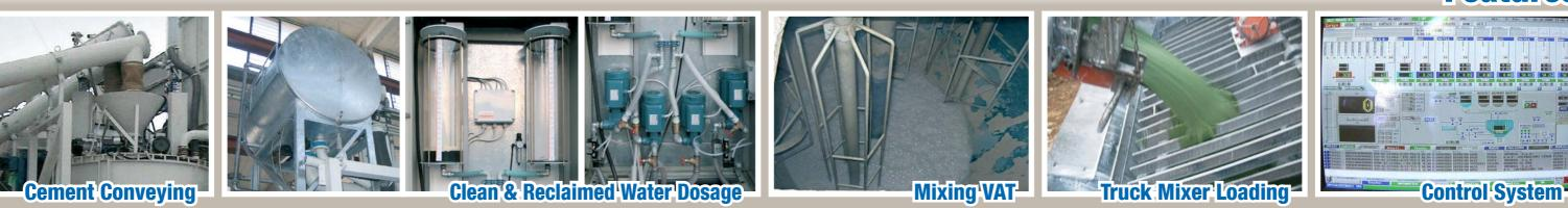
Two pipe systems are installed, one for conveying the cement paste to the truck mixer loading point and the other for recirculating the cement paste. Clean water holding tank is installed on top of the mixing vat to speed up the water dosage and automatic washing cycles.
